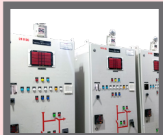
Control Relay Panels
